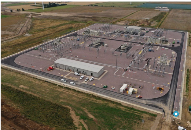
Image 2: Example of AIS site layout
