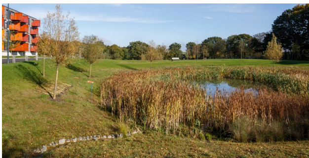
Image 23: xample of attenuation pond / Source: Essex SuDS design guide
